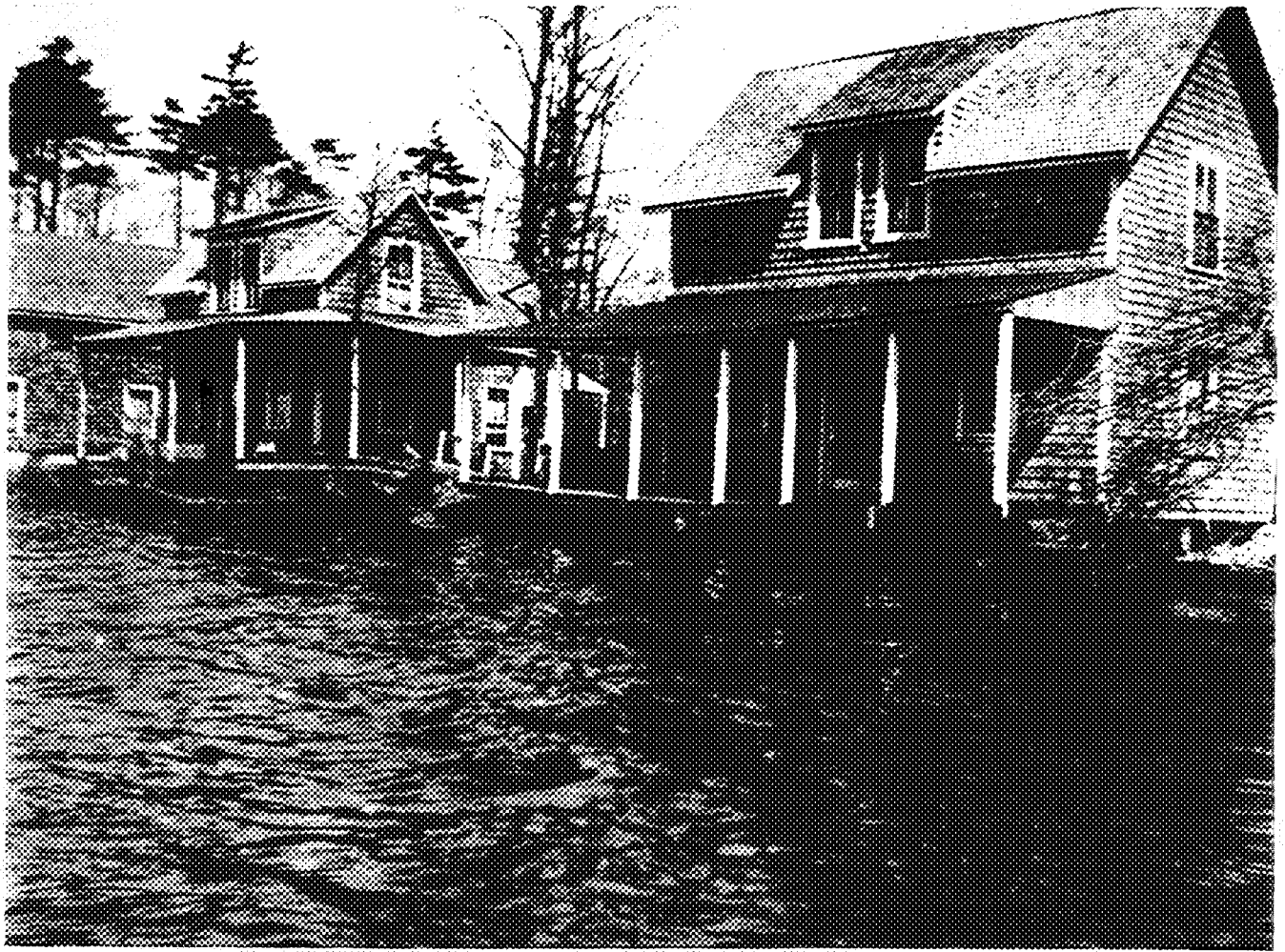
COTTAGES at Lake Assawompsett, 1920, damaged by ice and high water. (Photos courtesy of George Barden)
